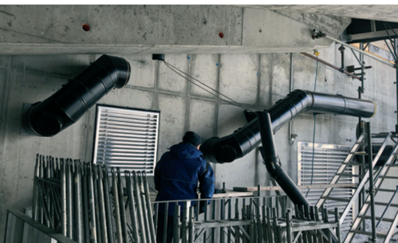
Installation of a stainless steel gas flue system from three emergency heat generators | Klein Matterhorn (3 883 m above sea level), Switzerland
