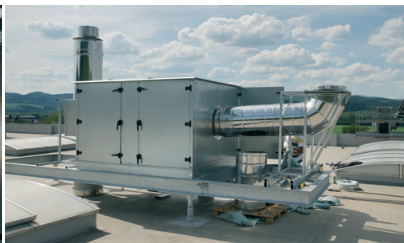
Installation of a stainless steel gas flue system from three emergency heat generators | Klein Matterhorn (3 883 m above sea level), Switzerland
